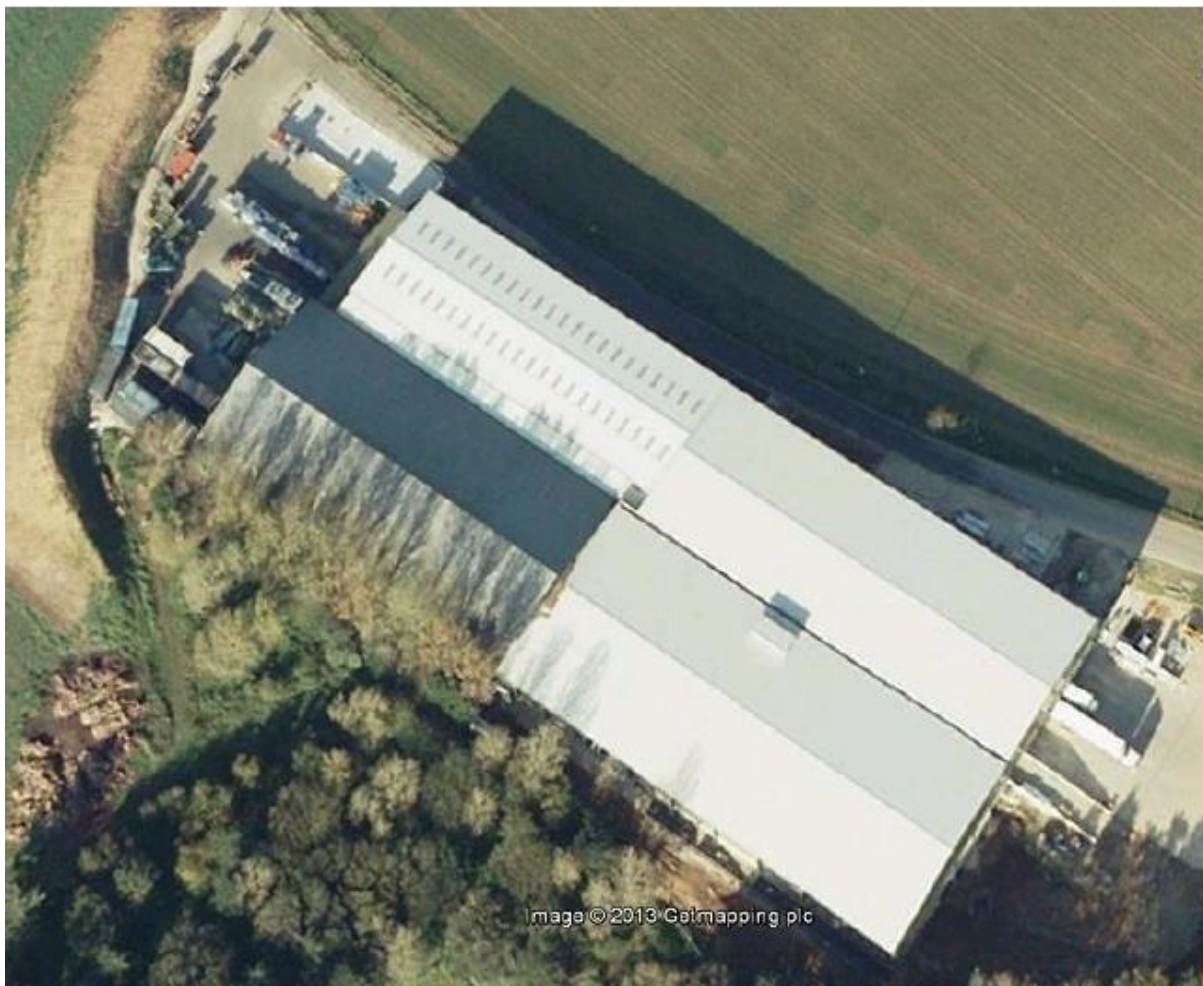
Figure 1 Aerial view of warehouse showing the original (aged) roof and the roofs of three further stages of extension and the large building footprint.
