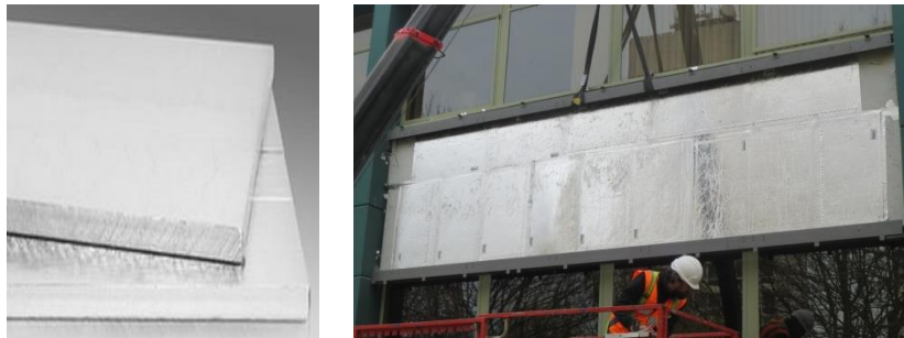
Figure 8. Image of a VIP and Final installation on-site
