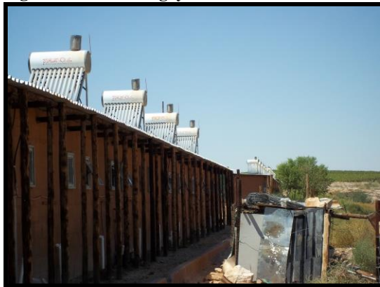
Figures 2 & 3: The geyser installations on worker housing units and the ‘donkey’ structure
