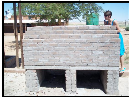
Figures 2 & 3: The geyser installations on worker housing units and the ‘donkey’ structure
