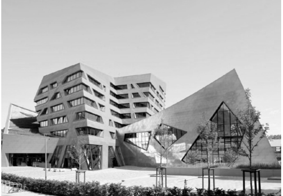
Central Building of Leuphana University. Image credit: Schüco International.
