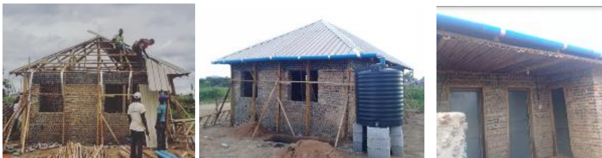
Figure 9: Roof Construction with rainwater harvesting
