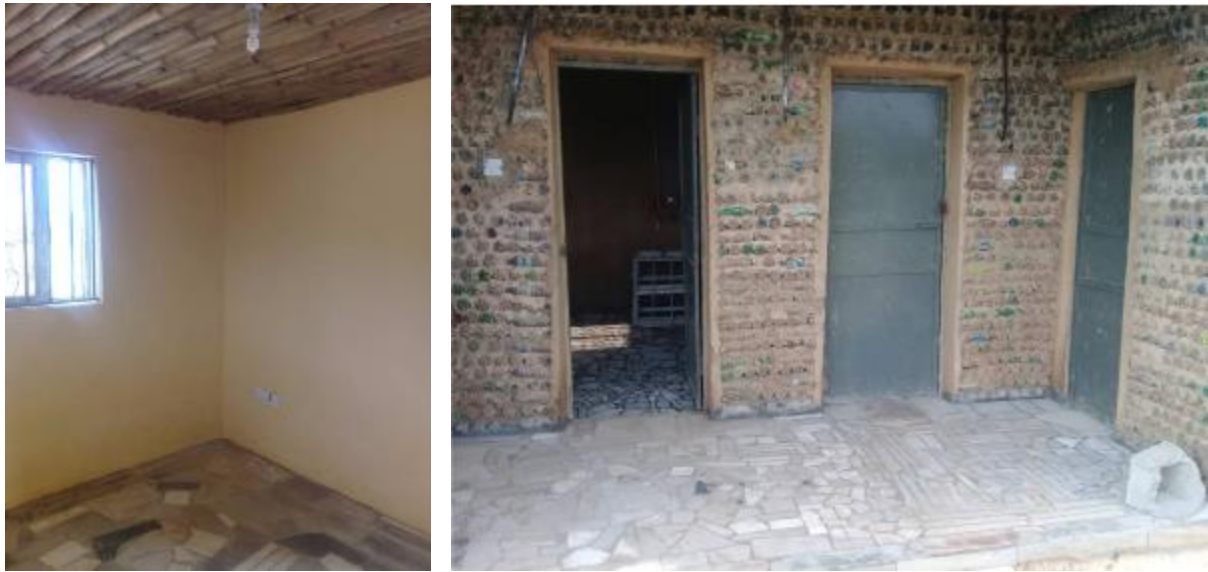
Figure 10: Plastered walls and finished floor.
