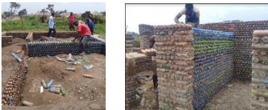
Figure 8: Plastic bottle Wall construction
