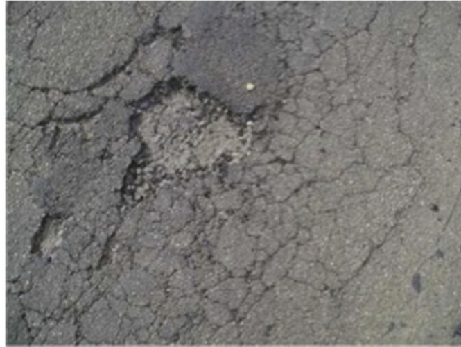
Fig. 1. Wear losses on pavements by aging effect.
