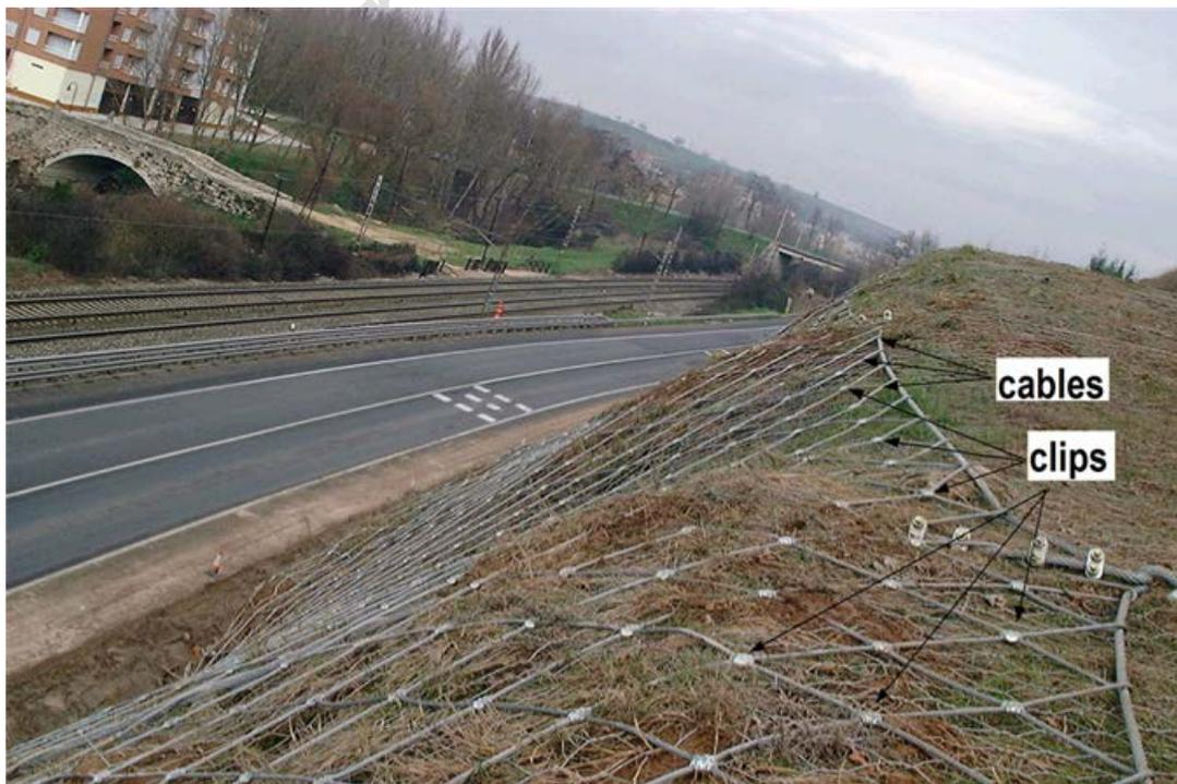
Figure 3: Actual application: cables and clips joints in a net over a road slope.
