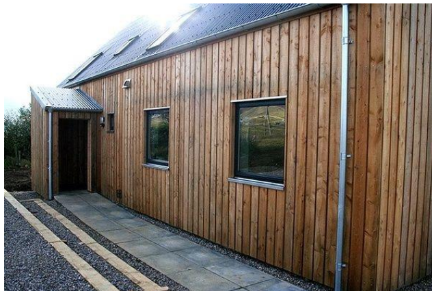
Figure 4 Vertical cladding (Cromartie Ltd, 2010)
