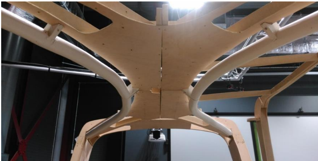
Figure 11.5 Handrails installed along the main Roof Structure
