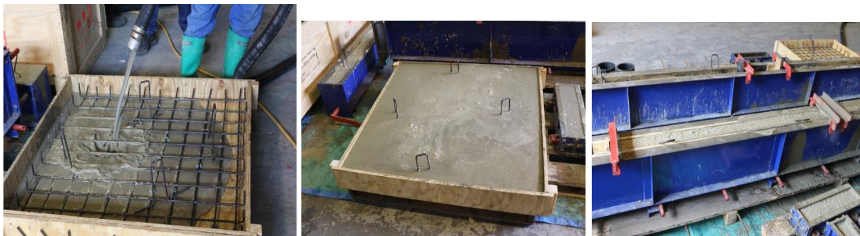
Figure 6: GEM-TECH material pumped into slab and beam moulds
