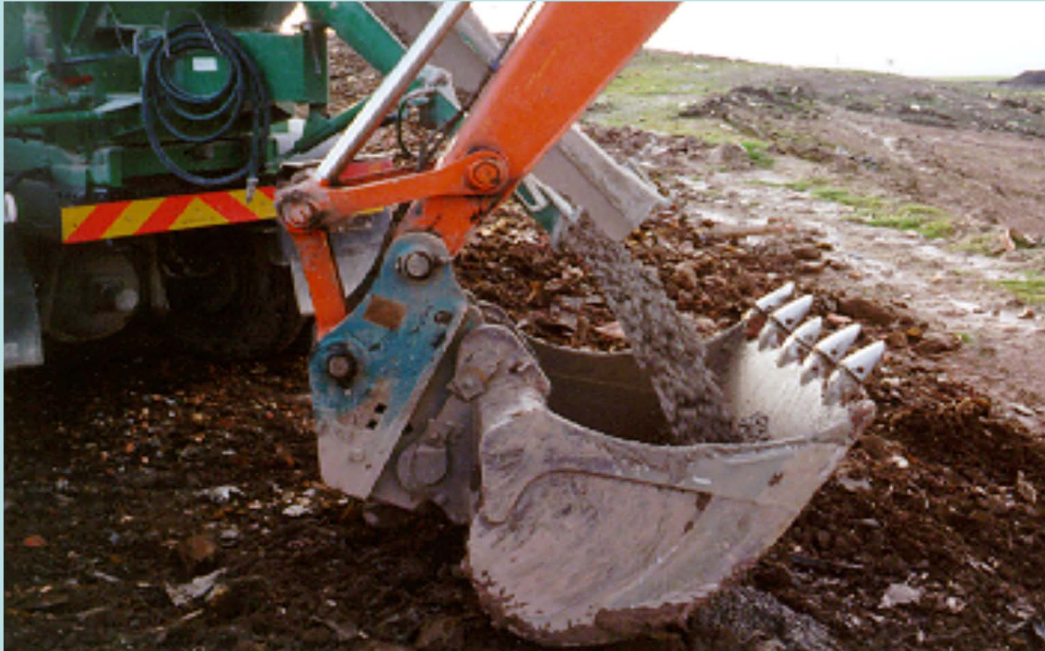
Concrete delivery to bucket
