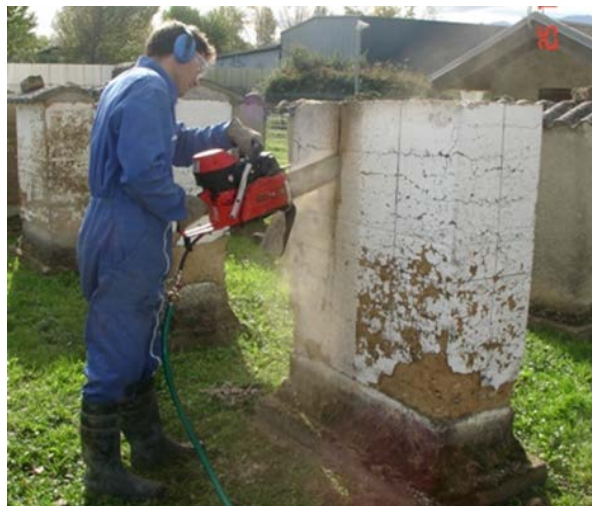
Figure 8. Cutting a wall with chainsaw.
