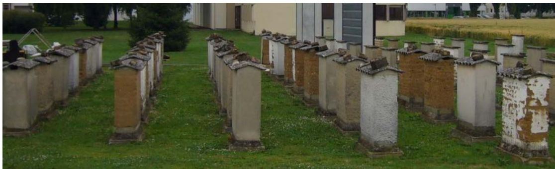
Figure 2. Rammed earth walls constructed and exposed for 22 years to natural weathering.
