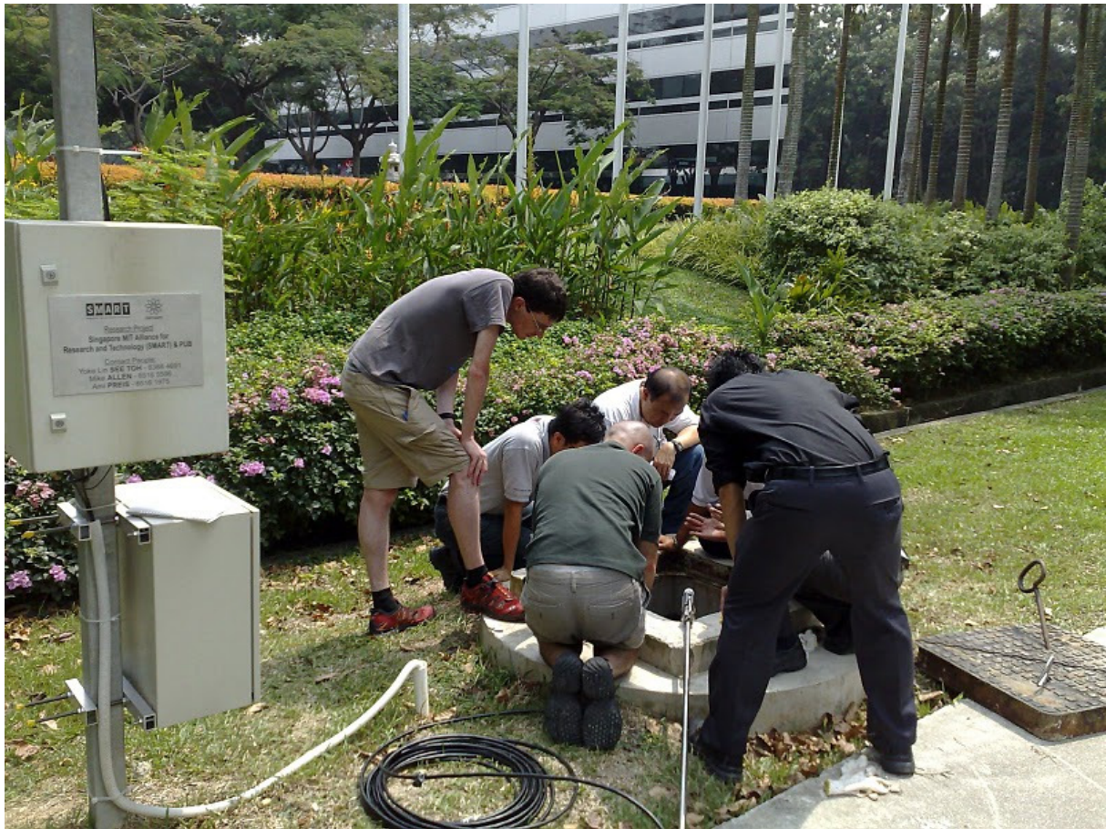
Figure 5.4: Debugging a WaterWiSe sensor node
