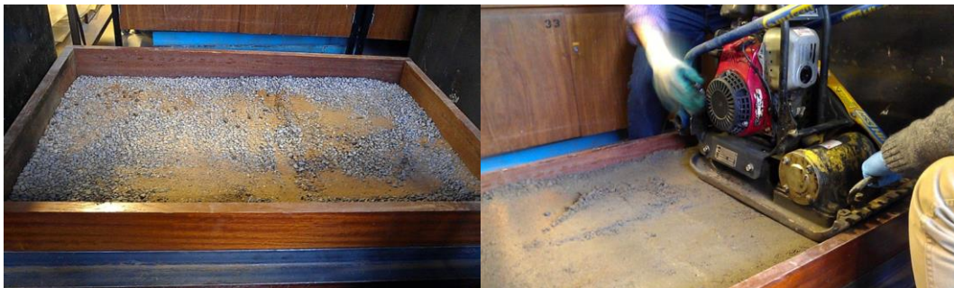
Figure 4.41 Foundation Preparation (a) Compacted Gravel (Left) (b) Cement Bound Material (CBM) Compacted with a Whacker Plate (Right)
