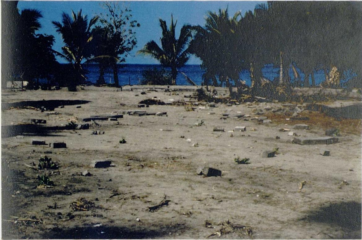
Plate 6. Concrete slabs transported from the foundation of a house by the tsunami at Nanganmepah, Nebe.
