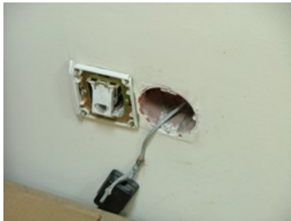
Figure 5.6: Electrical damage, Düzce State Hospital.
