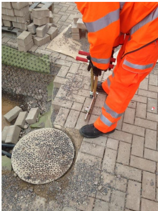
Figure 7.7 Removal of blocks on test bed
