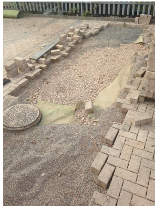
Figure 7.8 Test bed prepared for laying of blocks
