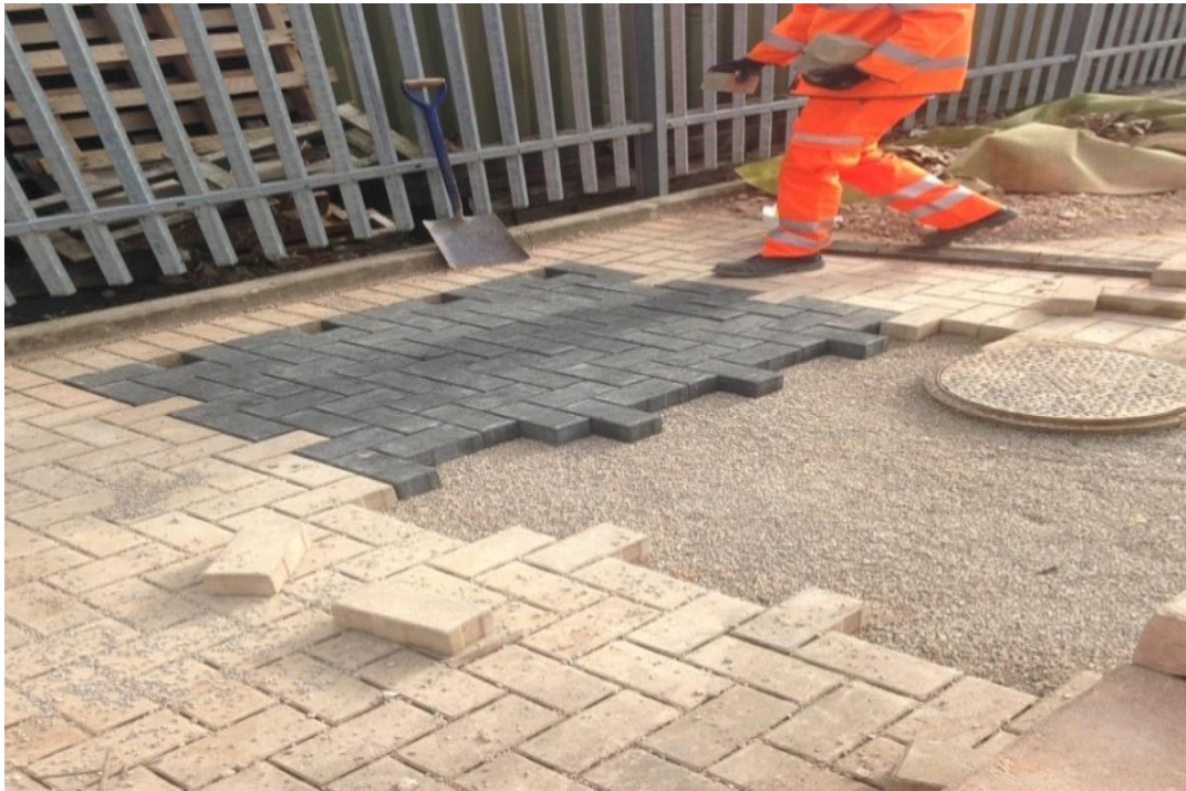
Figure 7.9 Blocks being laid on site
