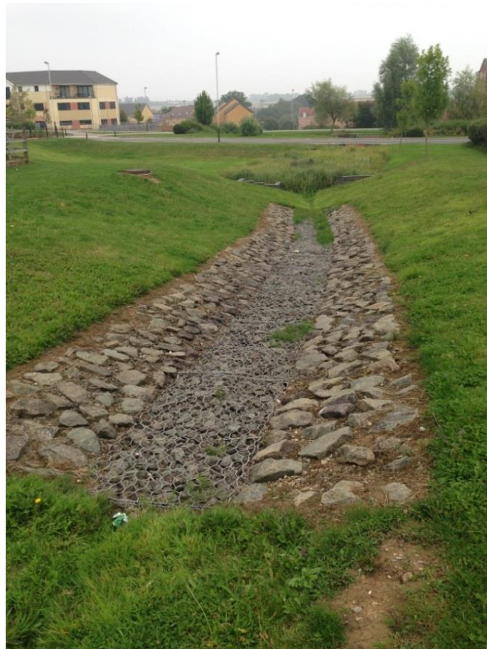
Figure 3-19 Rock-lined swale 1 with rip-rap on the base to limit erosion.
