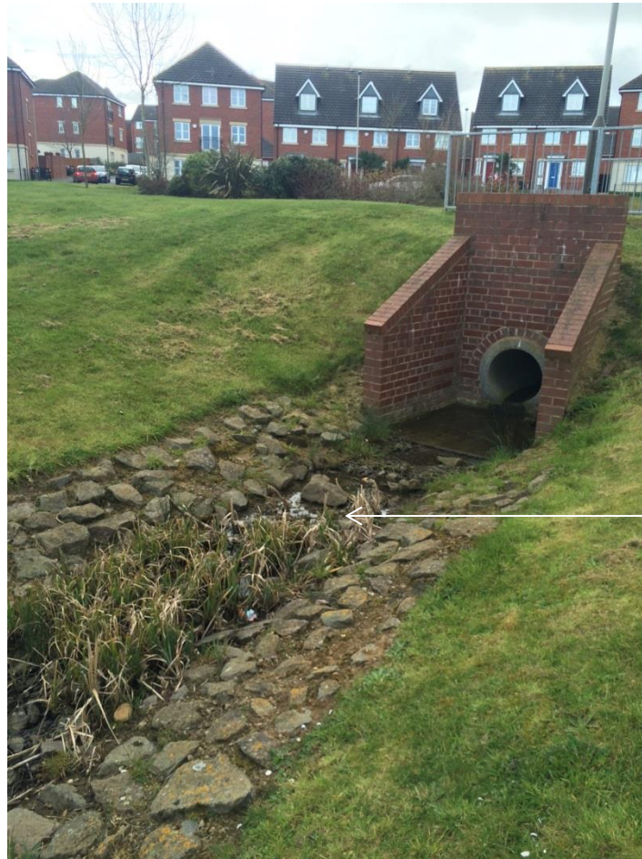
Figure 3-25 Site 2: Measurements were taken at the start of the rock lined swale.
