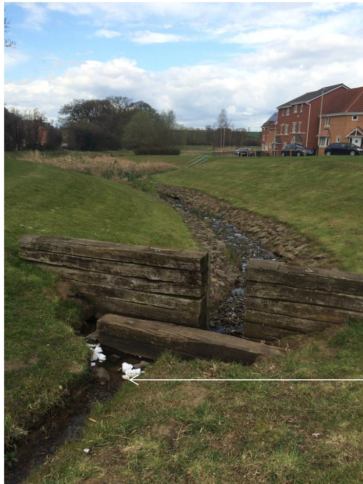
Figure 3-28 Site 5: Measurements were taken before the weir, at the end of the narrow channel. Note that the weir plate was stolen before measurements were taken, therefore the weir was not included in the final design in MicroDrainage ®.
