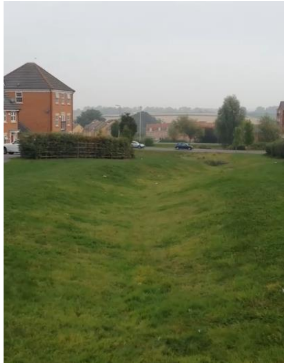
Figure 3-18 Swale 1 at Hamilton SuDS Management Train, Leicestershire.
