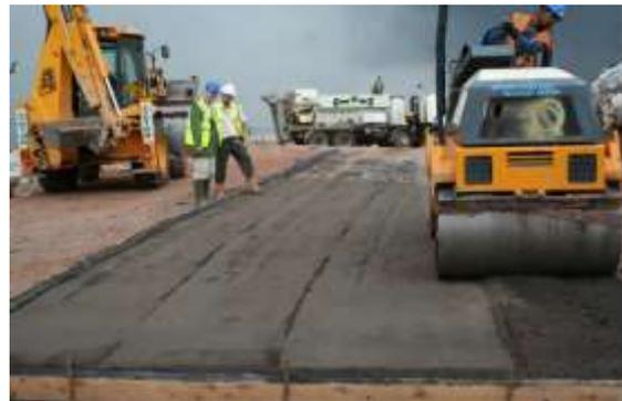
**Fig. 2.20b** Compacting the semi-dry paste
