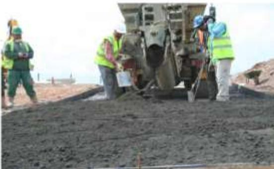
**Fig. 2.20a** Placing the semi-dry paste
