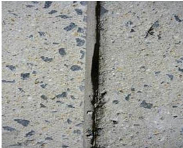
Figure 2-7: Medium level of joint seal damage (FHWA 2003).
