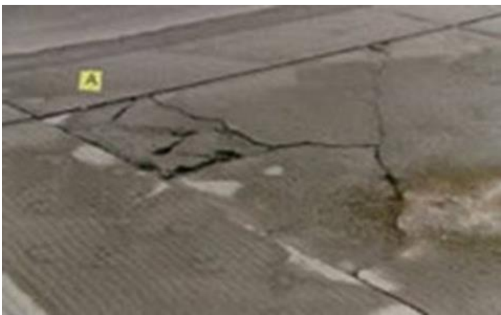
Figure 2-10: Contaminants in concrete pavement (The Constructor-Civil Engineering Home 2017).
