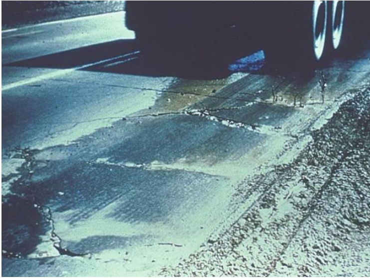
Figure 2-9: Water bleeding in concrete pavement (FHWA 2003).
