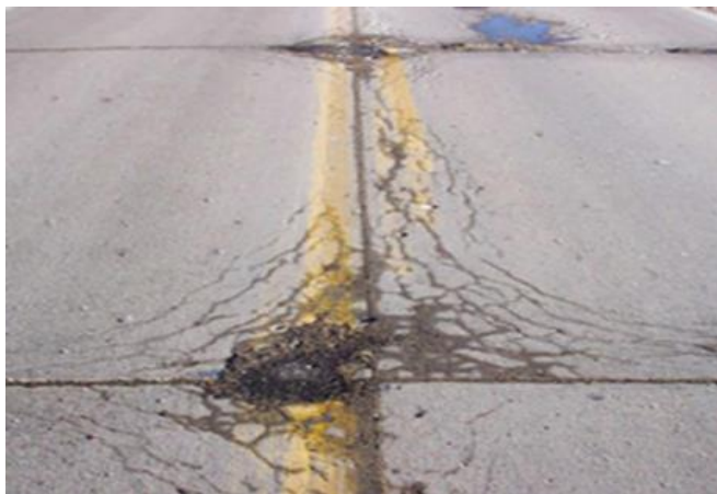
Figure 2-6: D-cracking in concrete pavement (Desta 2014).
