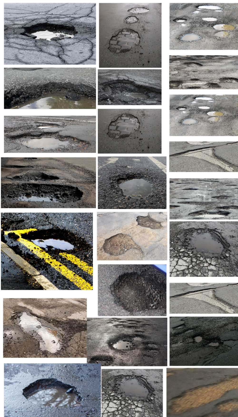
Figure 37 : Damaged road surface (DM02)
