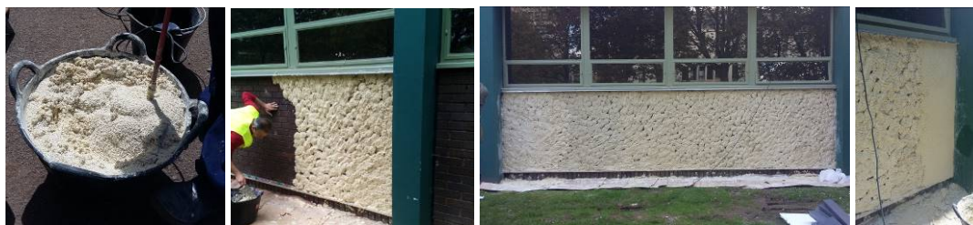
Figure 12: Installation of the aerogel mortar
