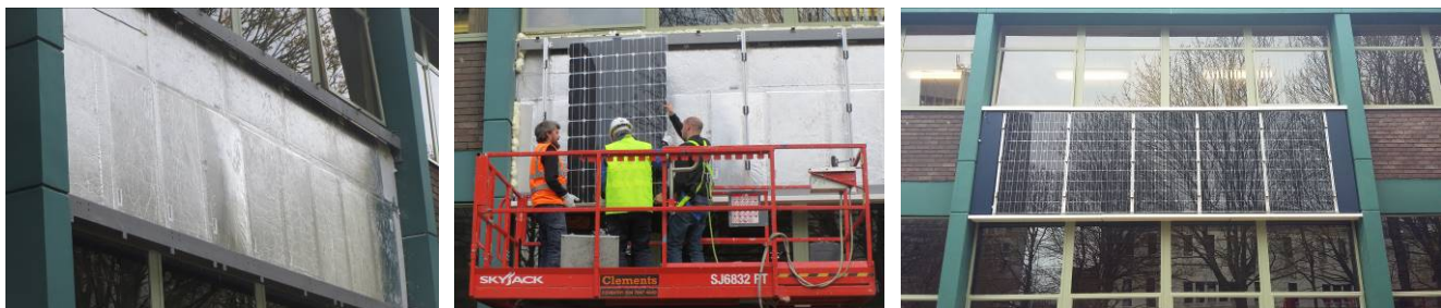
Figure 11. Installation of the ventilated façade
