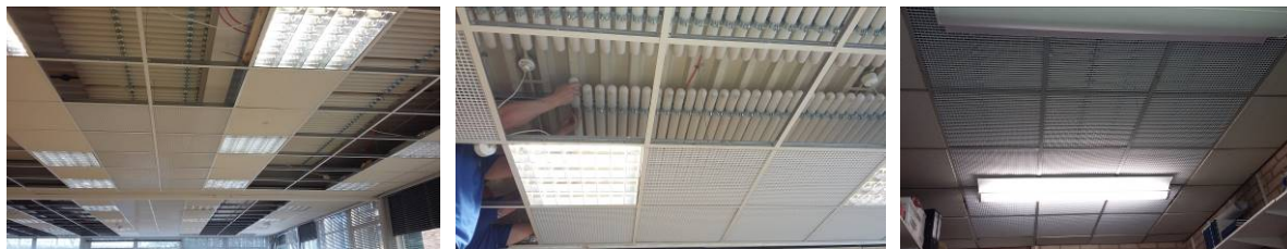
Figure 8: Installation of the PCM tubes
