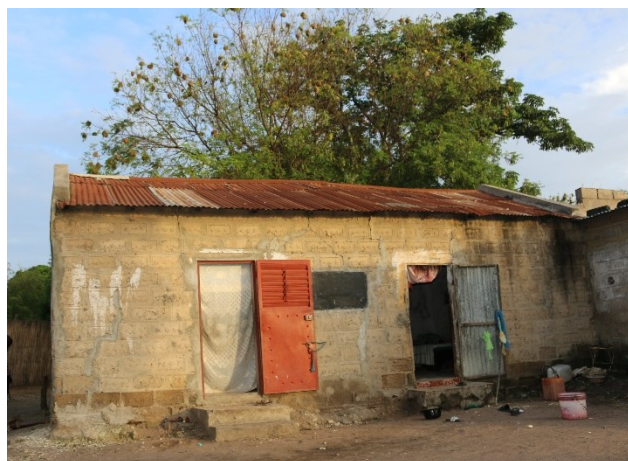
Figure 123. Brick, cement, and corrugated iron sheet construction in Ndiémane © Carla Sarrouy Kay 2019
