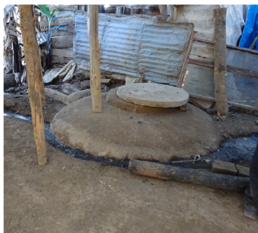
Fig. 1. Concrete fixed-dome biogas digester.
