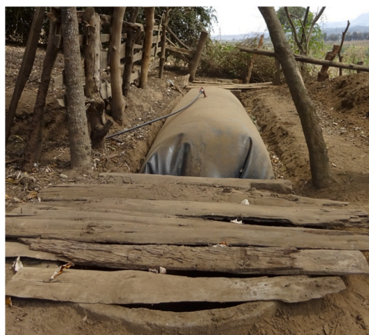
Fig. 2. Plastic bag biogas digester.
