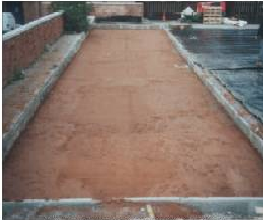
Compacted sand bedding layer below installation
