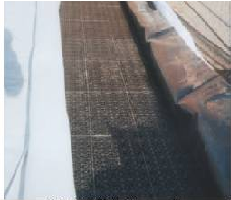
PERMAVOID™ Pad within geomembrane
