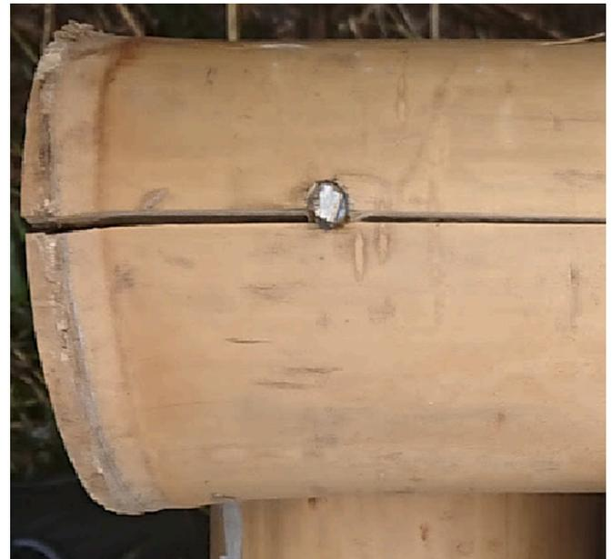
Fig. 2. Splitting in nailed connection (Coffee region, Colombia).
