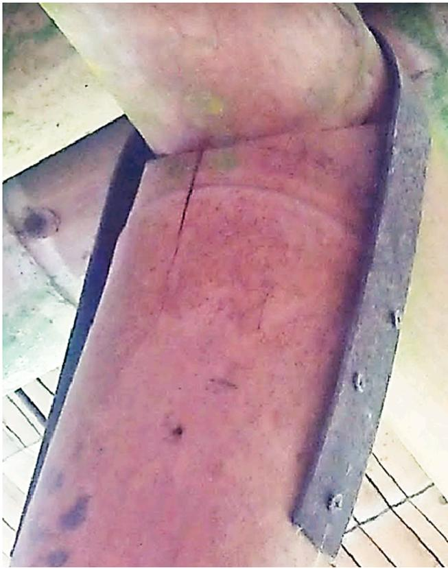
Fig. 3. Example of a screwed bamboo connection with metal plate (Coffee region, Colombia).
