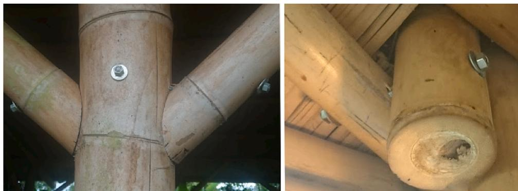
Fig. 1. Examples of bamboo bolted connections (Coffee region, Colombia).
