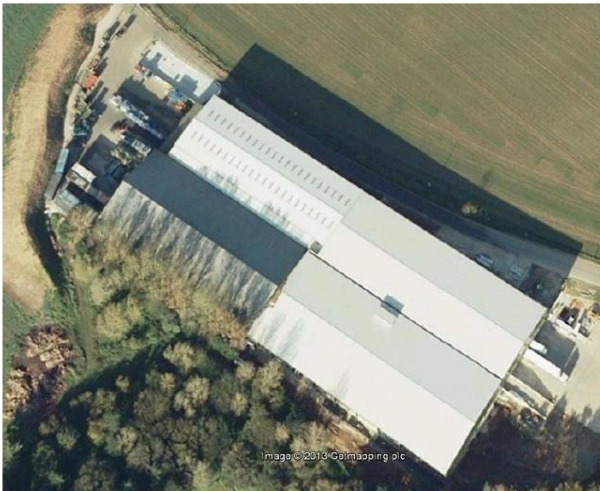
Figure 1 Aerial view of warehouse showing the original (aged) roof and the roofs of three further stages of extension and the large building footprint.
